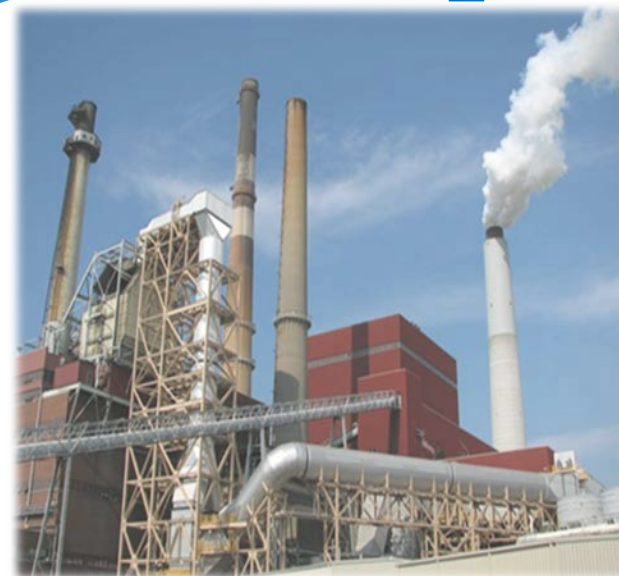
10-25 MWe Demonstration Unit (LG&E KU and DEDI)
