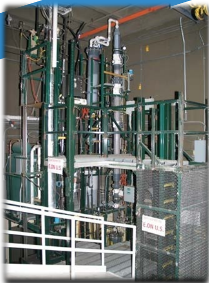
0.02 MWe (0.1 MWth) Pilot-scale Unit
